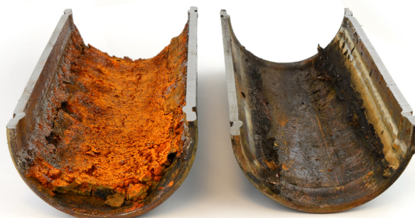
20 Month Pipe Test with Air
