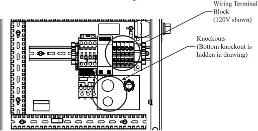
3. Depending on the voltage of the model (115V, 230V, 460V-Single or Three phase) follow the wiring diagram in this manual on page 39, or use the wiring diagram on the inside of the nitrogen generator cabinet door.
