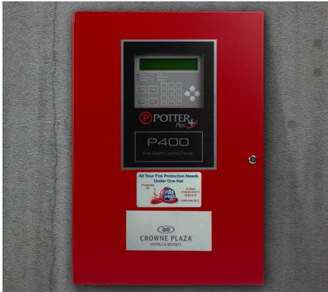
P400 panel. It was also very easy for them to incorporate firefighter telephones and elevator recall to ensure the safety of patrons as well as firefighters.
