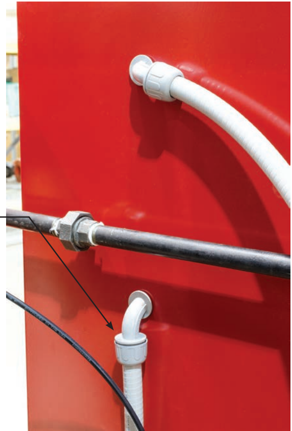
(Rear of Nitrogen Cabinet)
