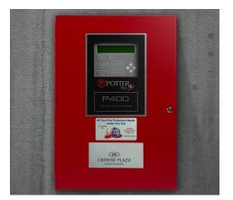
P400 panel. It was also very easy for them to incorporate firefighter telephones and elevator recall to ensure the safety of patrons as well as firefighters.
